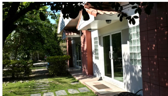
South side view of the building
